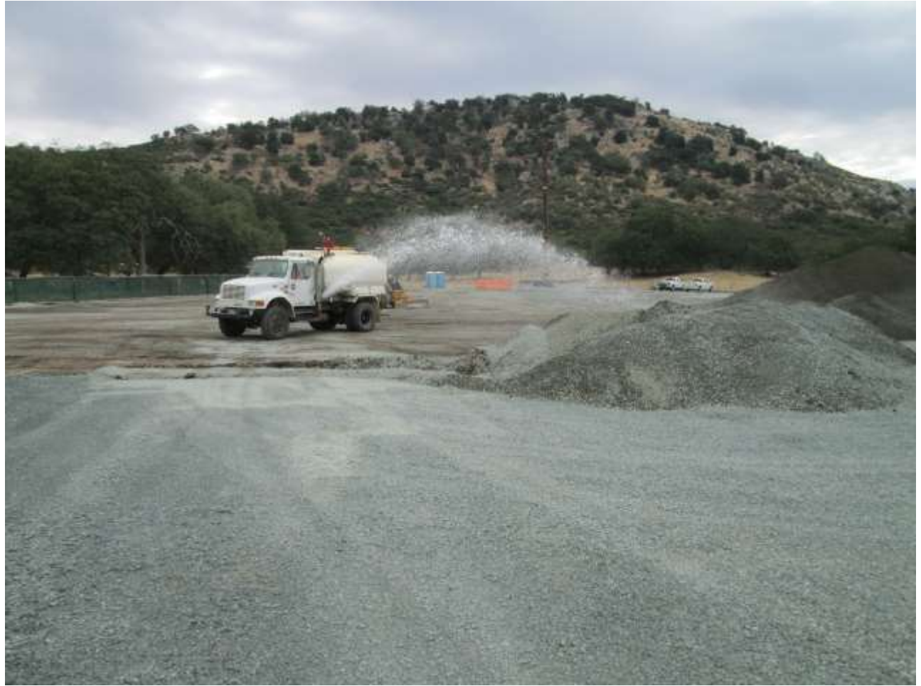
Photo 8: Crews were observed beginning to remove gravel from the Santa Ysabel Staging Yard. Water was applied to the gravel base layer prior to movement to ensure dust was minimized in accordance with MM-BIO-1.
